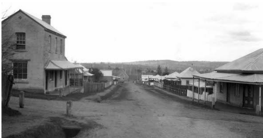
Wason St Milton, looking south from Charles St to Croobyar Rd. King (Legacy) House near left, Mudge’s workshops end of Wason St right side, and former Wesleyan Methodist Church in distance
