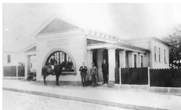
Milton Post Office single storey c.1900
